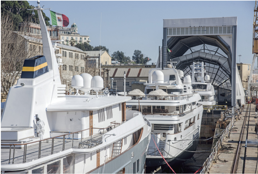
Left & below: The Amico dock and quayside facilities are perfectly positioned close to Genoa city centre.
