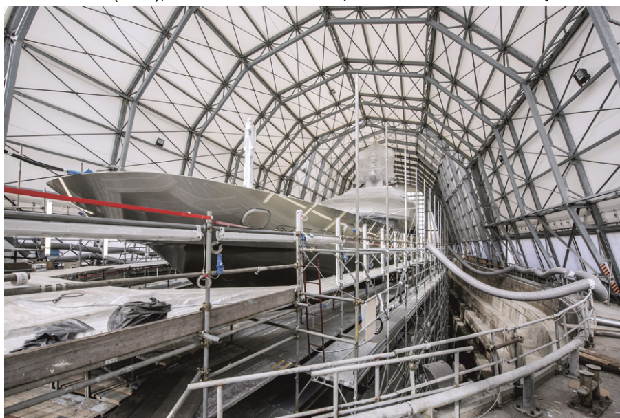
Amico's covered air-conditioned dock is a very recent investment.
